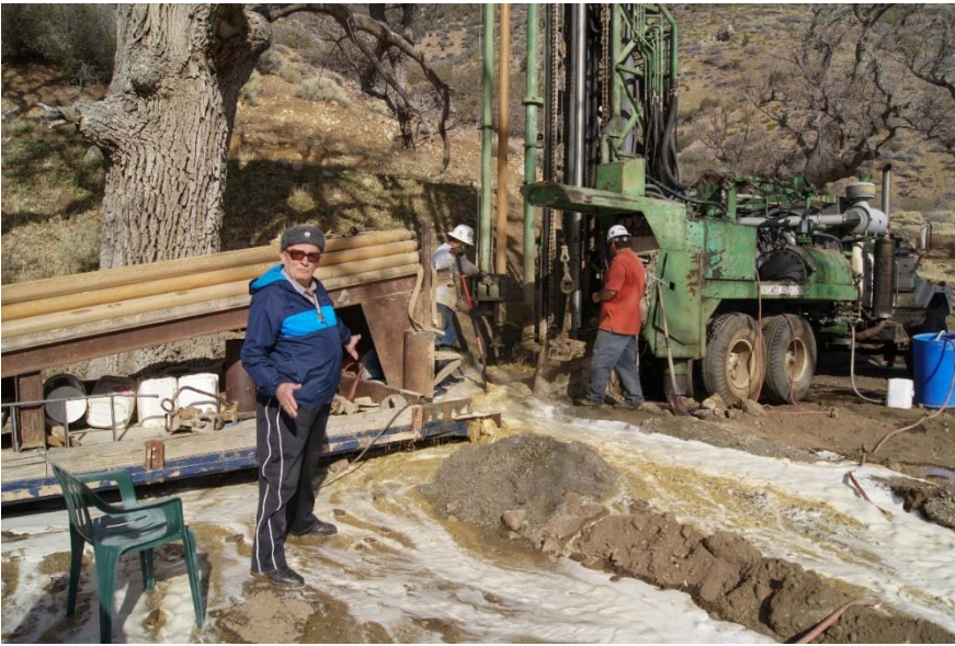
Pal drilled two test boreholes he called the Garlock Project on the Garlock fault, at a 6,000-foot elevation in the Tehachapi's above the Grapevine in California. It is estimated this site will produce 1,000 GPM per-well on land thought to be unproductive.
